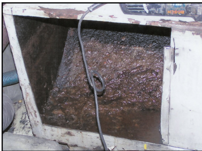
Tank with first front section removed, revealing extent of the problem
