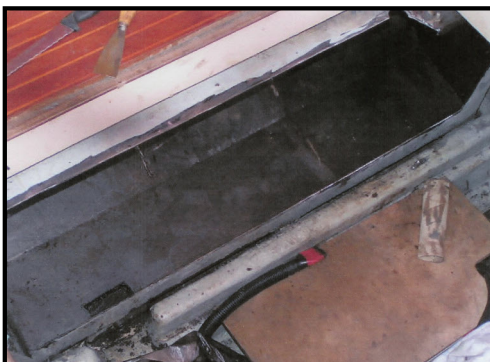
Tank cleaned and scraped prior to painting
