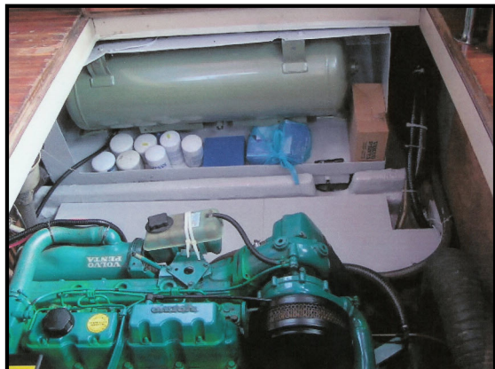
New fuel tank with storage space below
